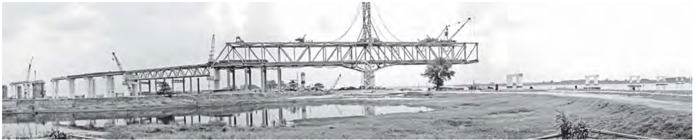
Construction of Ayeyawady Bridge (Nyaungdon) in progress.—MNA
