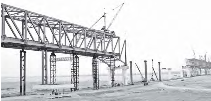
Photo shows completion of installation of steel truss of the bridge on Letpanchepaw bank.—MNA
