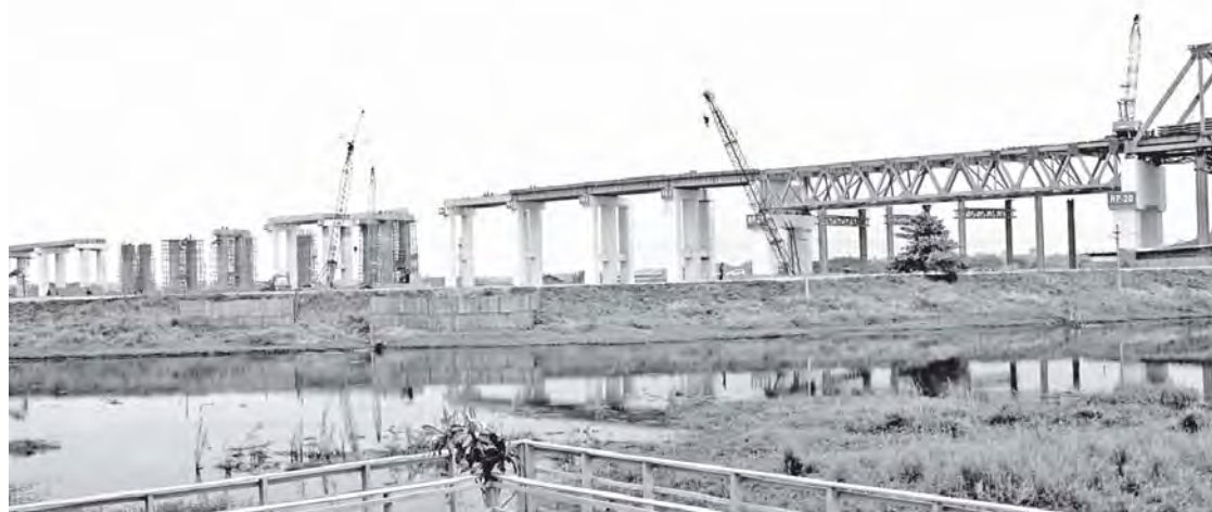
Progress in construction of Ayeyawady Bridge (Pakokku).—MNA
