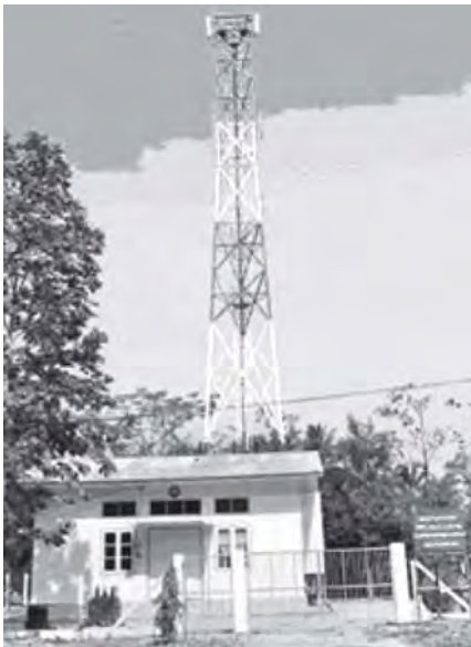
GSM station at 7th-Mile in Kawthoung.
