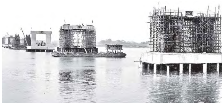
Progress in construction of piers of Ayeyawady Bridge (Nyaungdon).
