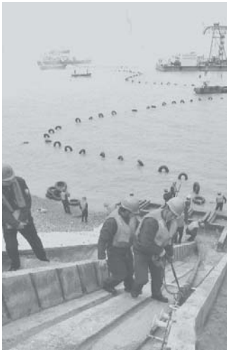
Workers drag a submarine cable onshore in Chengsi Island, Zhoushan City, east China's Zhejiang Province, on 16 March, 2011. XINHUA
