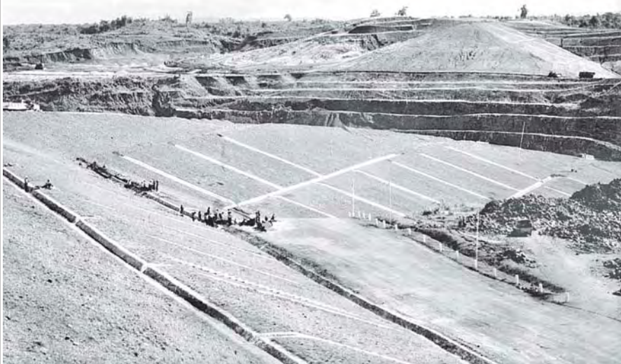
A dyke under construction in Kanyin Dam Project.
