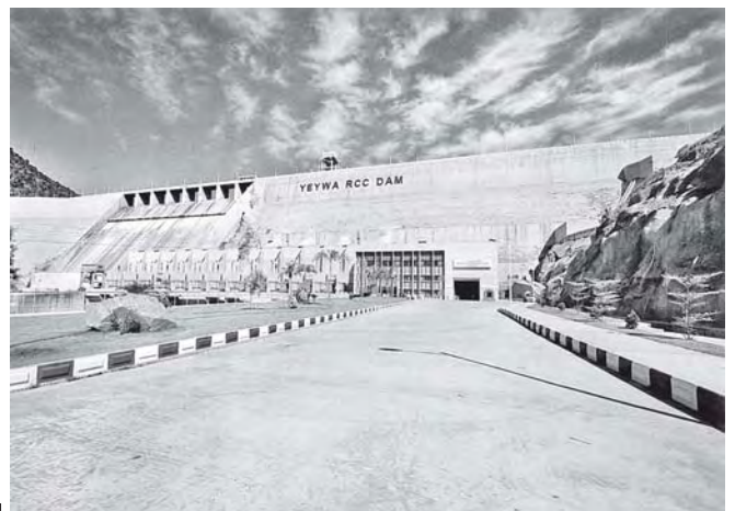
Yeywa Hydropower Plant and RCC Dam.
