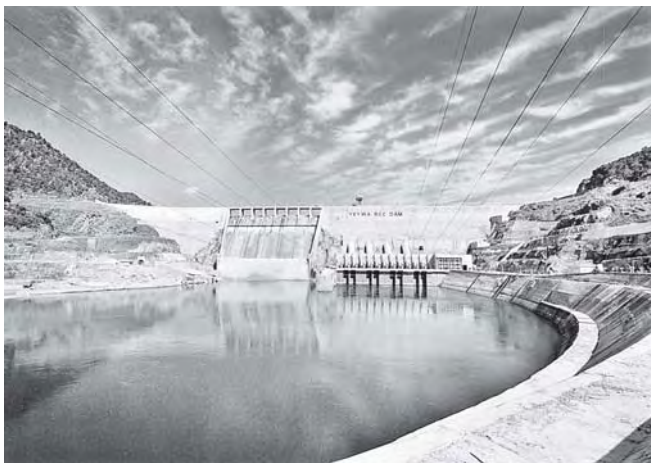
The RCC dam and the outfall channel of the plant.
