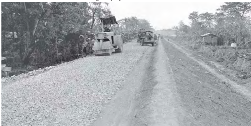
Placing of gravel on embankment road in progress in Thongwakyun.
