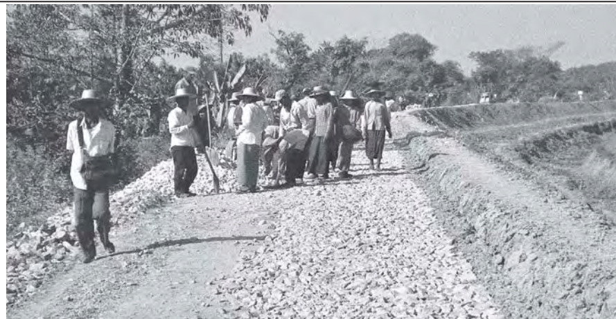
Workers seen at placing of gravel on Thongwakyun embankment road.
