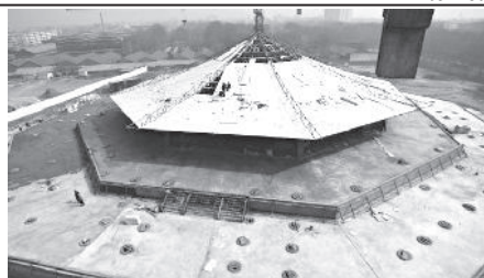
Photo taken on 23 Feb, 2011 shows the under-restoration Mingtang, an octahedral architecture in China's Tang Dynasty style, at Sui and Tang Dynasties Relics Protection Park in Luoyang City, central China's Henan Province.—XINHUA
