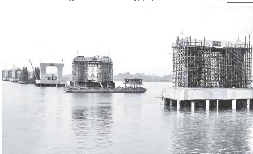
Photo shows piers of Ayeyawady Bridge (Nyaungdon).
