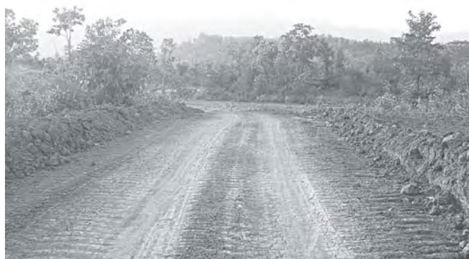
Photo shows progress of Ayechantha-Thitkyitaing Inter-Village Road.
