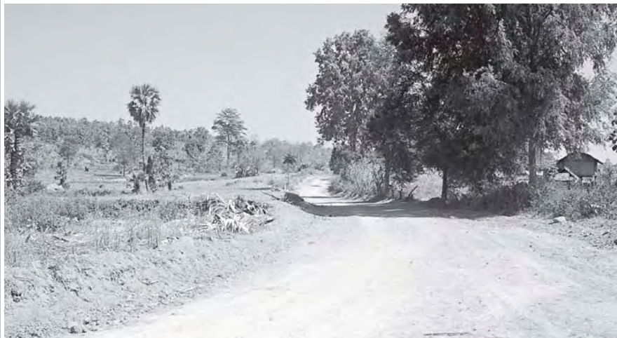
Photo shows progress of Kyetyin-Gaungbwa-Letpan Inter-Village Road.
