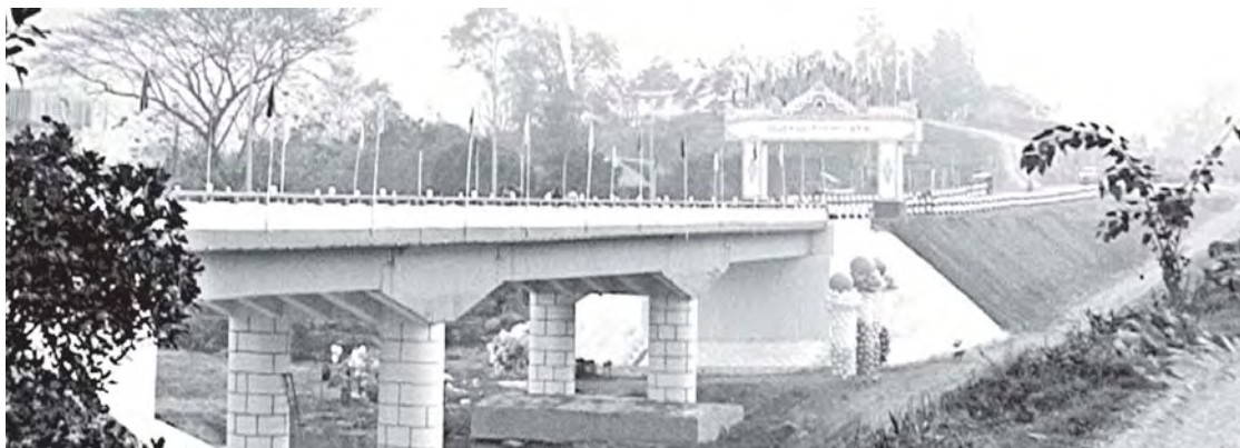
Pyinyaung Bridge on Meiktila-Taunggyi-Kengtung-Tachilek Road.—MNA
