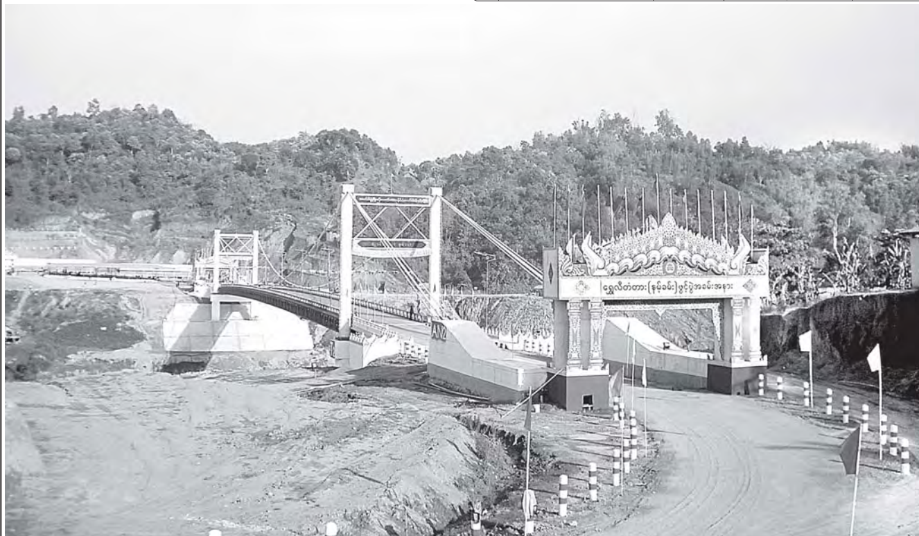
Photo shows Shweli Bridge (Namkham).
