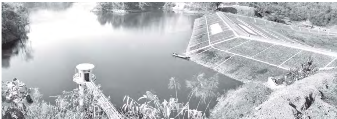
Pyaingchaung Dam stores water for irrigation and local consumption in Kyauktaw Township of Rakhine State.
