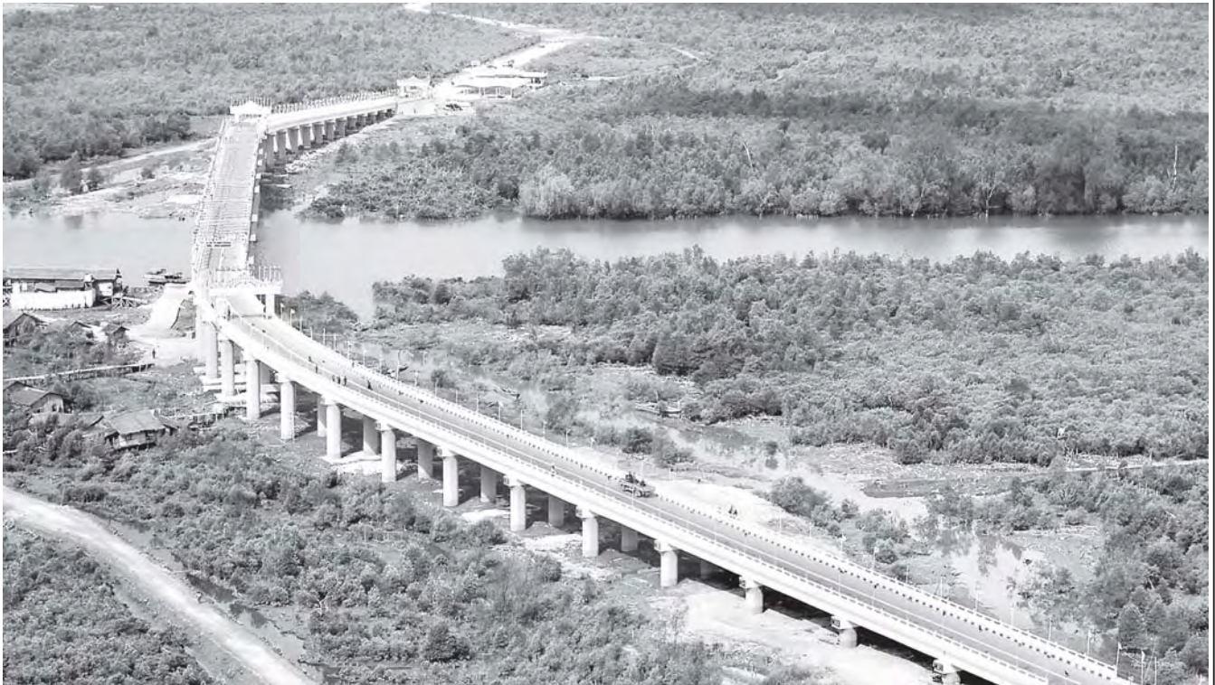
A bird's eye view of Minkyaung Bridge on Maei-Kyaukpyu Road Section built by the government in Yanbye Township of Rakhine State after 1988.
