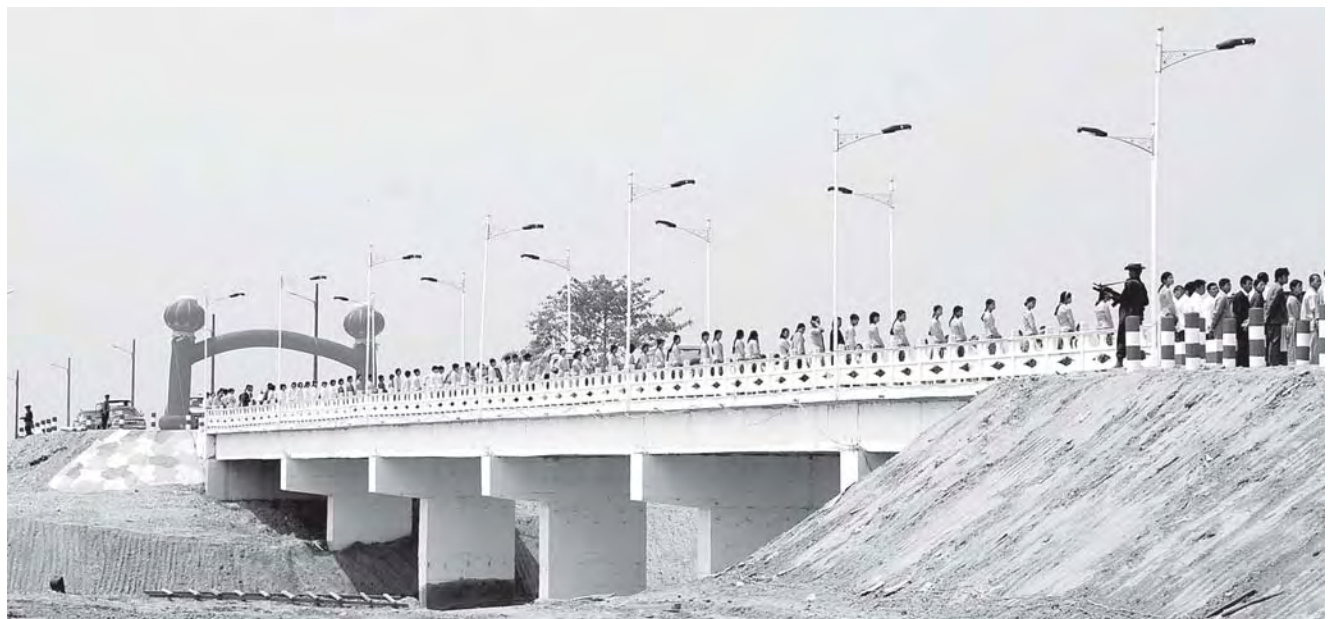
Warazup Bridge No. 2 on Myitkyina-Namti-Tanai Road.
