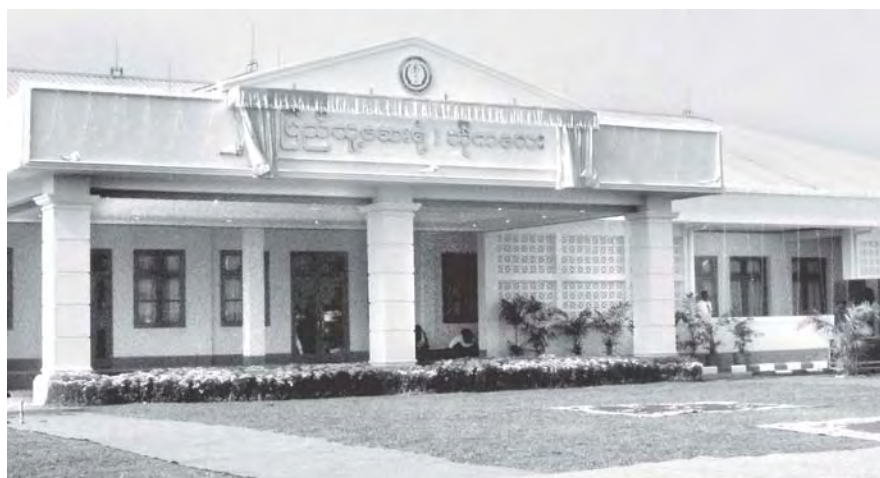
New People's Hospital (100-bed) in Bogale Township.
