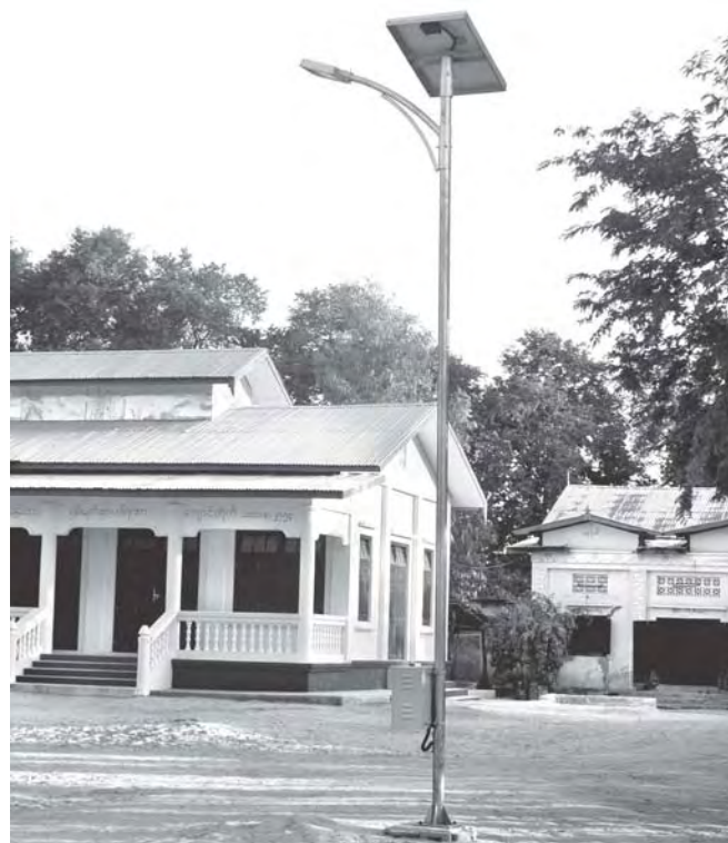
A solar lamp post installed with solar panel, bulb and energy control system in Ywathaya Village.
