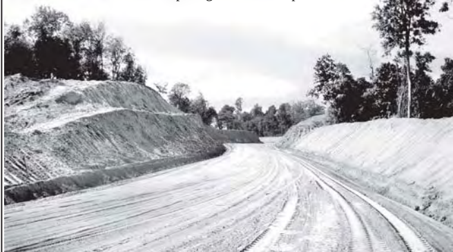
An expanded earthen section of Koebin-Thagaya Road.
