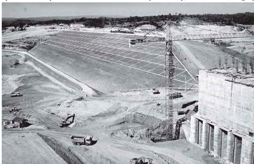
Earth work of Kyee-Ohn Kyee-Wa Multi-Purpose Dam Project is being undertaken with the use of machinery near hydro power station.
