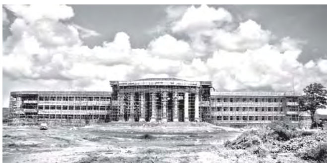
University of Computer Studies (Loikaw) under construction.
