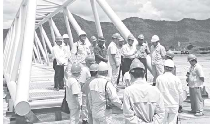
Minister U Lun Thi views installation of pipeline crossing Myitnge River of Myanmar-China Crude Oil and Natural Gas Pipeline Project near Kywenapha Village of Patheingyi Township.—ENERGY
