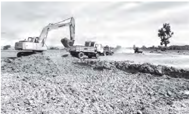
Heavy machinery raising the lower bund of Tanilale lake.
