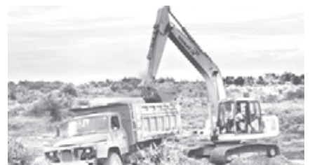
A tipper lorry and a backhoe at work to upgrade road sections in Tanai Township.
