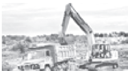
A tipper lorry and a backhoe at work to upgrade road sections in Tanai Township.
