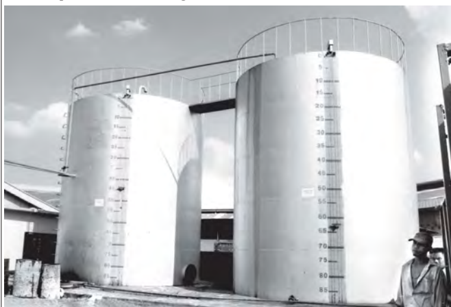
Photo shows two tanks that store quality soya bean oil before being packaged in Shwepyitha Industrial Zone.
