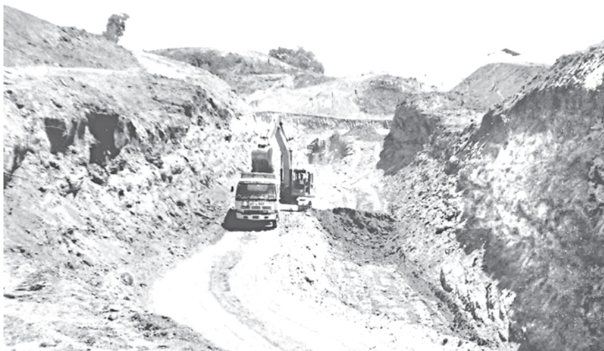
Heavy machinery cutting a hill to build spillway of Mokkha Dam.
