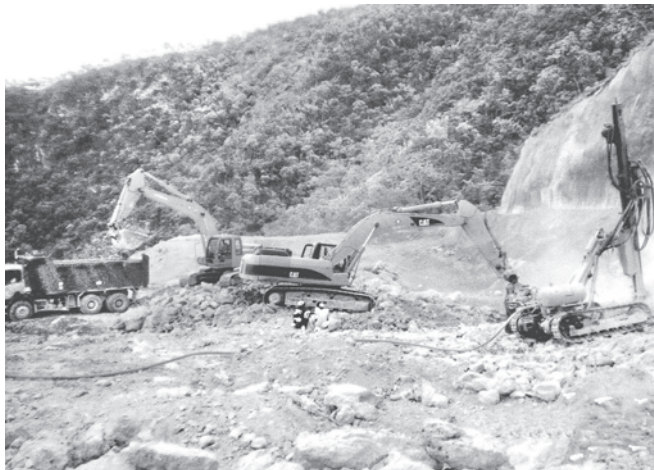
Works for constructing regulating lake in progress.
