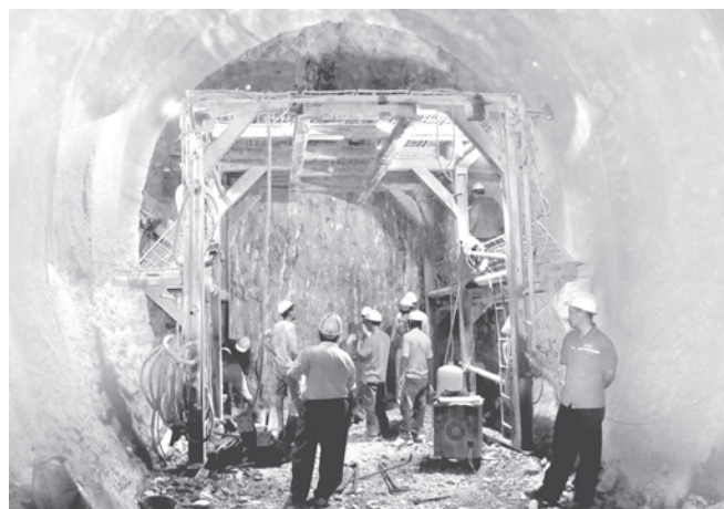
Construction of upper wall in inner main water intake tunnel.
