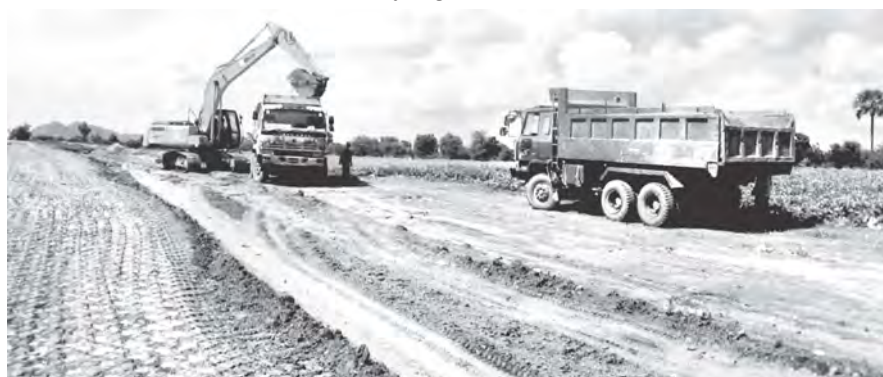
Earth work of Pathein-Monywa Asphalt Road being undertaken with the use of heavy machinery.
