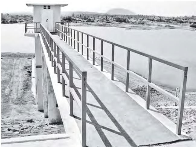
Embankment and control tower seen at Gwaygyo Dam in Yesagyo Township.
