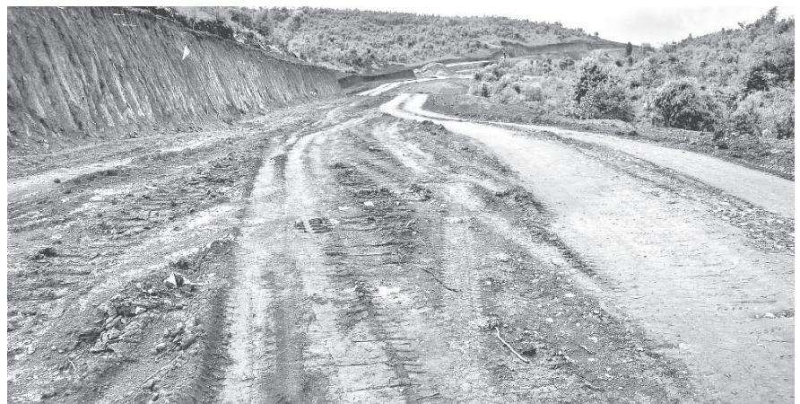
A road section near Medaw Village awaits gravelling.
