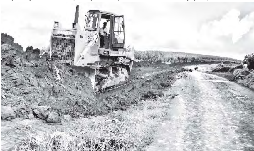
Groundwork is nearing completion near Nyaunggon Village.
