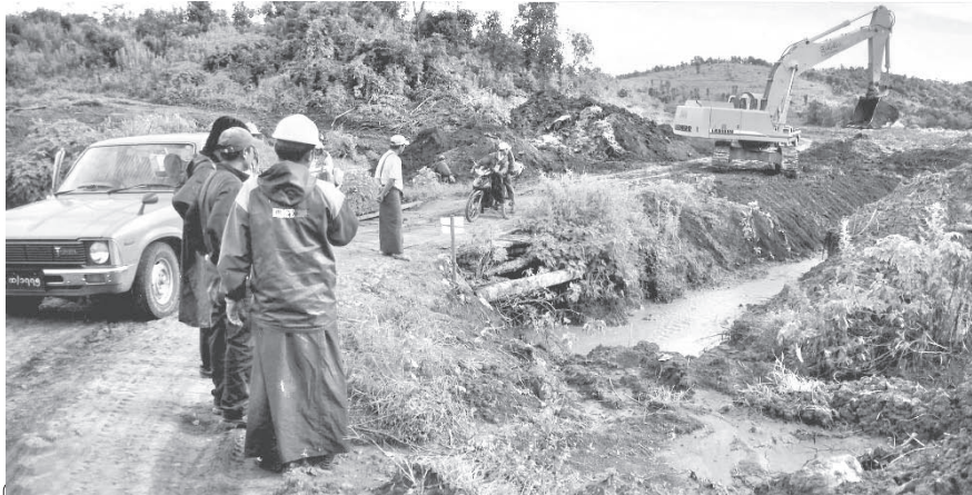
A unit of heavy machinery carrying out groundwork near Naungpein Village.
