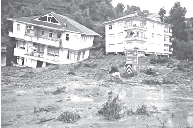
A man walks past a house tilted sideways after landslides and floods triggered by heavy rains swept through a Gundogdu near Turkey's Black Sea coast on 27 Aug, 2010. People were killed when the landslide collapsed homes in Gundogdu, in the tea-growing Black Sea province of Rize.
