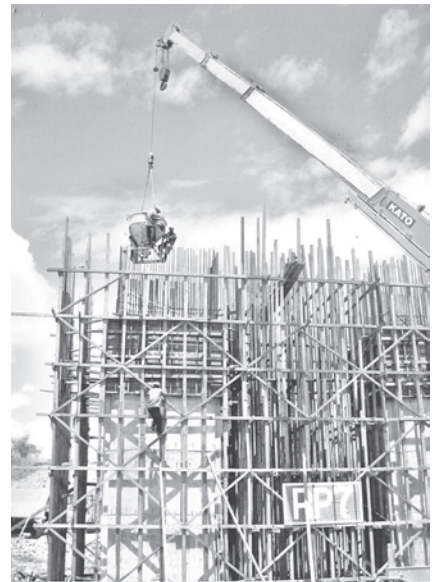
Construction of posts for Yadanatheinga Bridge on the bank of Singu.
