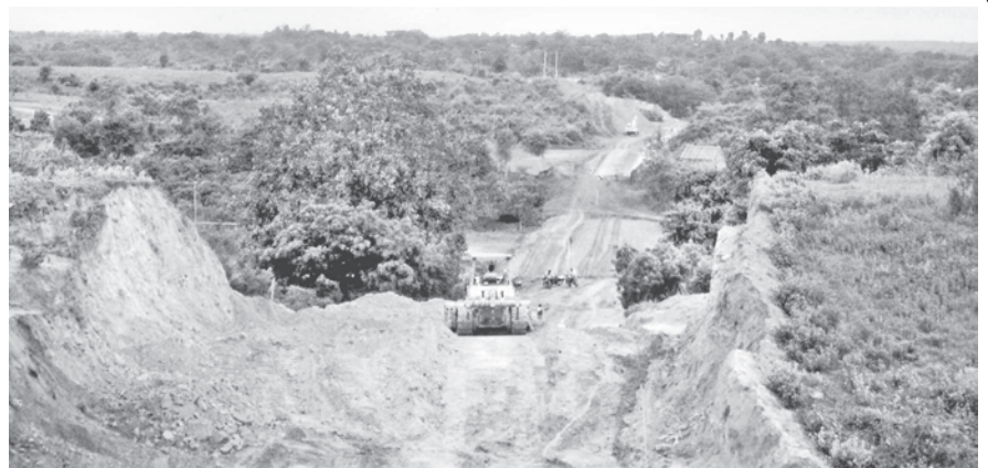
Construction of approach road on the side of Kyaukmyaung.
