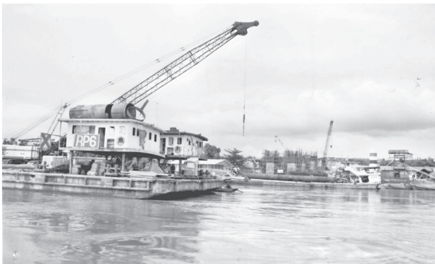
Ayeyawady Bridge (Yadanatheinga) under construction.
