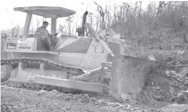
Land preparations for construction of Natkar Dam.
