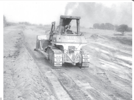
Heavy machinery at work.
