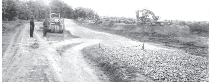
Minhla-Seinkantlant-Myochaung-Peinzalok-Bantbwagon-Penwewagon road section is under construction with the use of heavy machinery.
