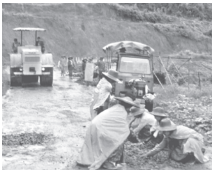
Taungup mountain pass under repair with labour and heavy machinery.
