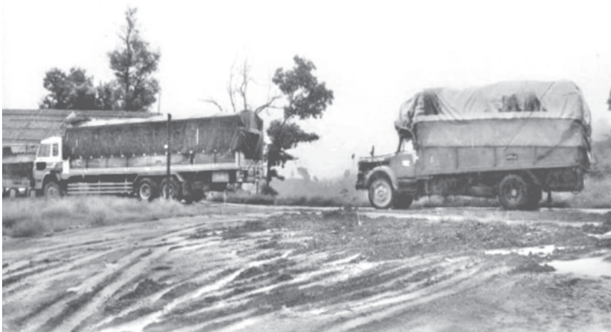
Two trucks loaded with goods on Taungup mountain pass, an all-weather facility.
