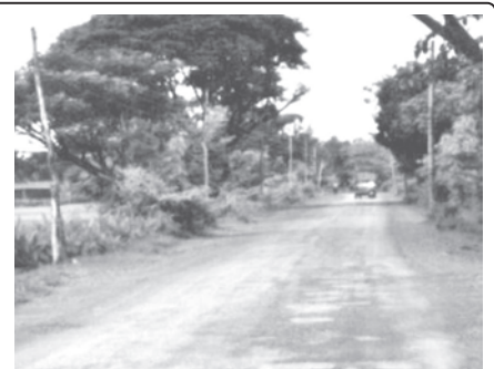
Taungup-Seikkan gravel road has been upgraded to a tarred one by Naylathitsar Co.
