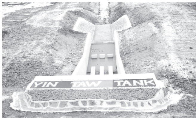
Southern feeder canal of Yintaw Tank irrigating 2,400 acres of farmlands.
