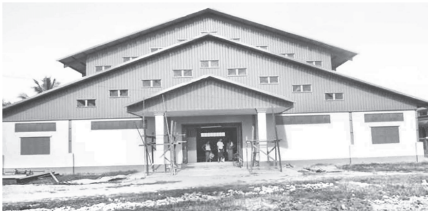
A gymnasium built in Bogale.
