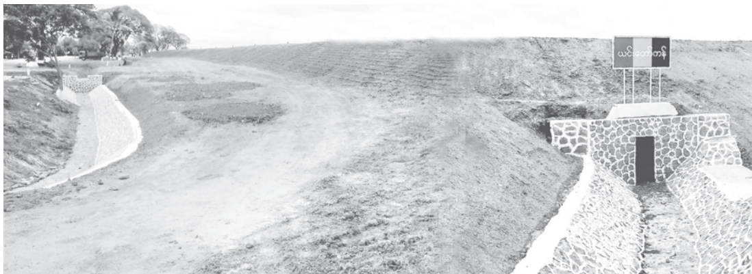
Photo shows the drain, feeder canal and bund of Yintaw Tank.
