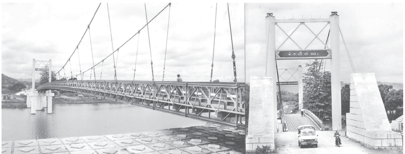
Mezali bailey suspension bridge built across Mone Creek in Pwinbyu Township.
