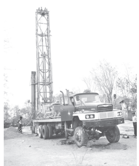
Water Resources Utilization Department sinking a tube-well near Ayethaya Village of Pyawbwe Township.
