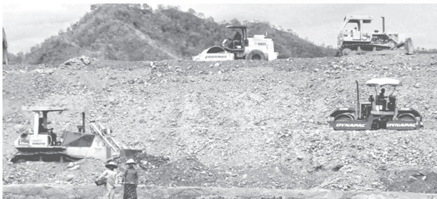
Heavy machinery at work at Myogyi Multi-purpose Dam Project.
