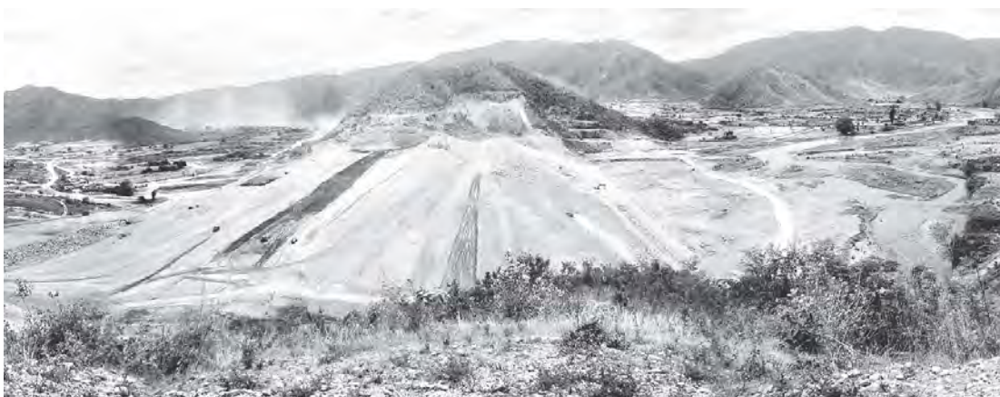
Main embankment is under construction at Myogyi Multi-purpose Dam Project.
