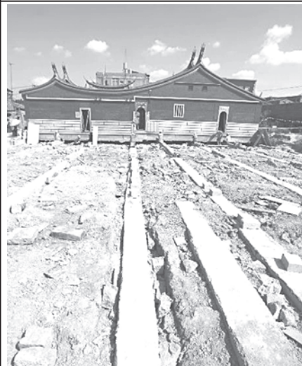
Workers move the Chaidamen ancestral hall by using jacks in Jinjiang City, southeast China's Fujian Province, Aug. 8, 2010. Because of the Shiji Road expanding project of Jinjiang City, the whole Chaidamen ancestral hall, with a history of over 300 years and a weight of 362 tons, was being lifted and moved 30.8 meters eastward. The move will be completed until Monday afternoon. XINHUA
