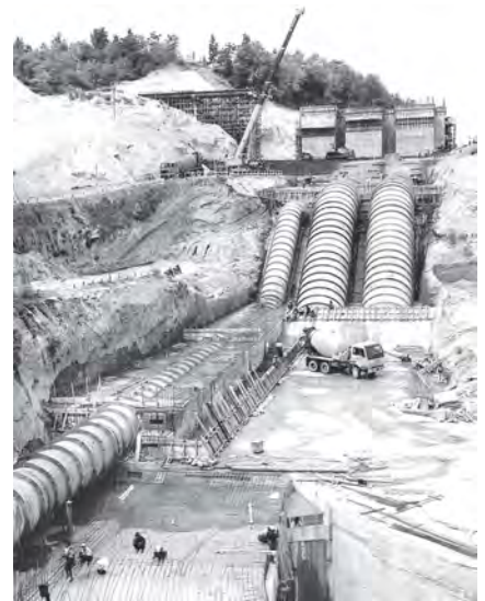
Installation of penstock steel pipelines in progress.
