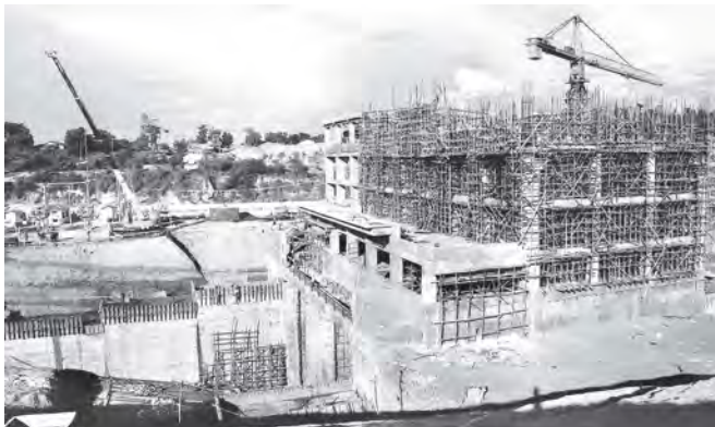
Power station is under construction to generate 74 megawatts.
