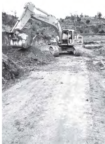
Medaw-Naungpein road section on PyinOoLwin-Mogok Road being constructed by Ayeya Shwewah Co in PyinOoLwin District.
