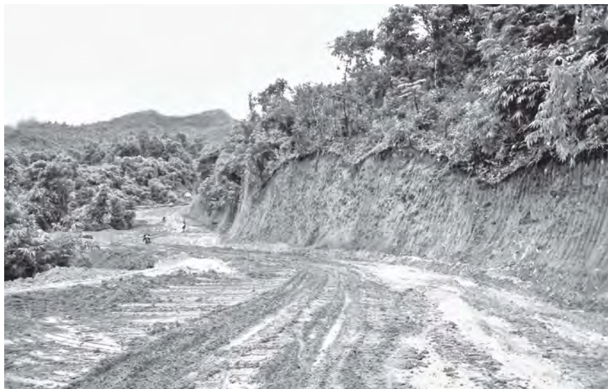
New PyinOoLwin-Mogok Road expended to 34 feet wide earth road on a hill in Legyi Village of Mogok Township.
