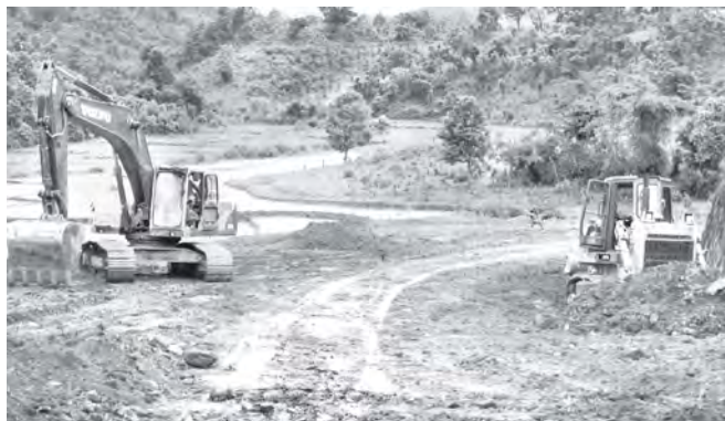
Progress of PyinOoLwin-Mogok Road construction project seen with heavy machinery.
