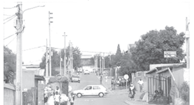
The theft of electric cables for their copper wire has led to power cuts in South Africa.—INTERNET
