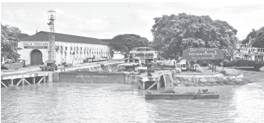
Dalla Dockyard seen on Yangon River.
