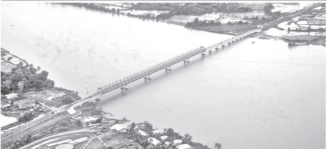
Photo shows an aerial view of Yazudaing Bridge No. 1 across Yazudaing River which is an invaluable transport facility for local people in Mawlamyinegyun Township, Ayeyawady Division.—MNA
