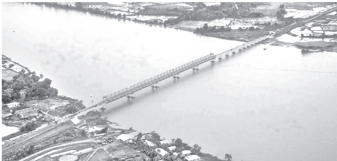
Photo shows an aerial view of Yazudaing Bridge No. 1 across Yazudaing River which is unvaluable transport facility for local people in Mawlamyinegyun Township, Ayeyawady Division.—MNA
