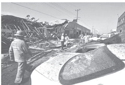
Los Angeles city fire fighters survey damage after a suspected natural gas explosion at a welding shop collapsed part of the building and hurled two workers into the street, killing one and leaving the other in critical condition on 30 July, 2010, in Los Angeles.—INTERNET
