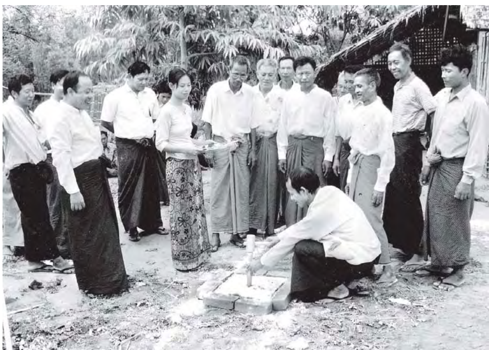
Head of Monywa Township Information and Public Relations Department U Aung Swe Win and a townselder lay corner stones for construction of a library in Zetaw Village, Khawaekyin Village-tract in Monywa Township, Monywa District on 26 June, 2010.
