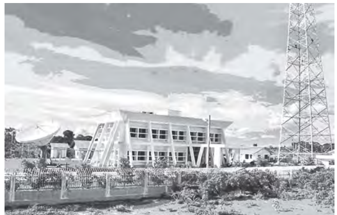
CDMA station in Taungdwingyi, Magway Division, indicates regional communication progress.
