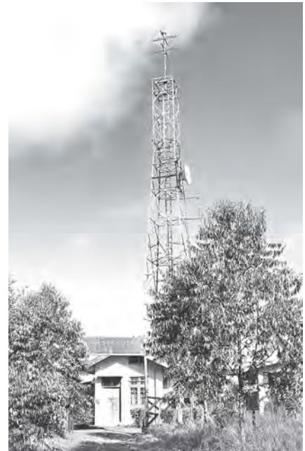
TV retransmitting station of Falam in Chin State.
