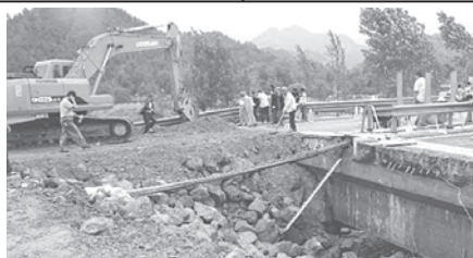
Workers repair the flood-destroyed Fuzhou-Yinchuan expressway in the section of Shanyang County, northwest China's Shaanxi Province, on 25 July, 2010. — XINHUA
