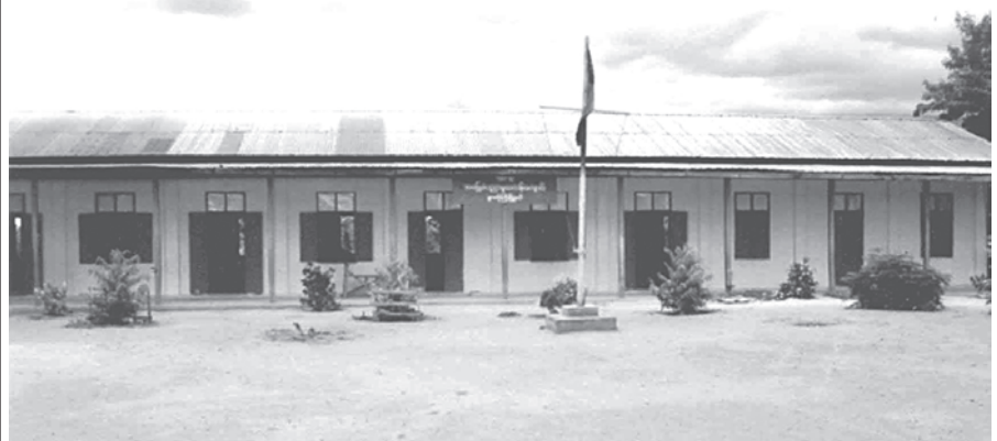
New school building of Thaminbe Village Basic Education Primary School.
