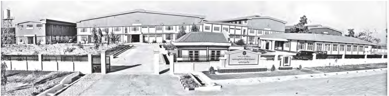
Import-substitute Hydro Turbine and Generator Factory.
