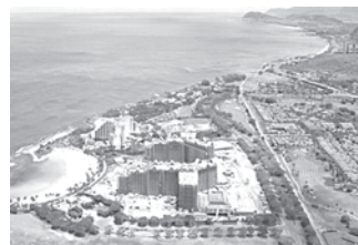
This undated photo provided by Disney Enterprises, Inc shows Construction on Aulani, a Disney Resort & Spa in Ko Olina, Hawaii. The resort is scheduled to open on 29 Aug, 2011 and features two 15-storey room towers, an expansive pool and garden area, spa, restaurants and access to a 9-acre lagoon and Ted Robinson designed 18-hole championship golf course.
