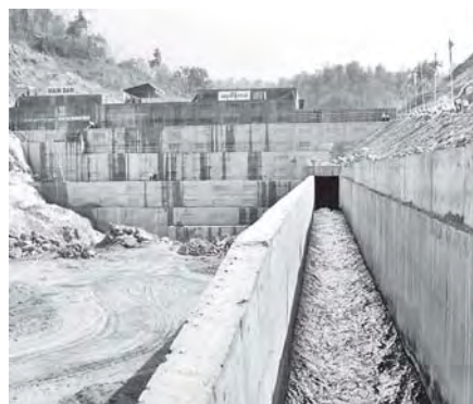
Nancho Hydropower Plant is under construction.
