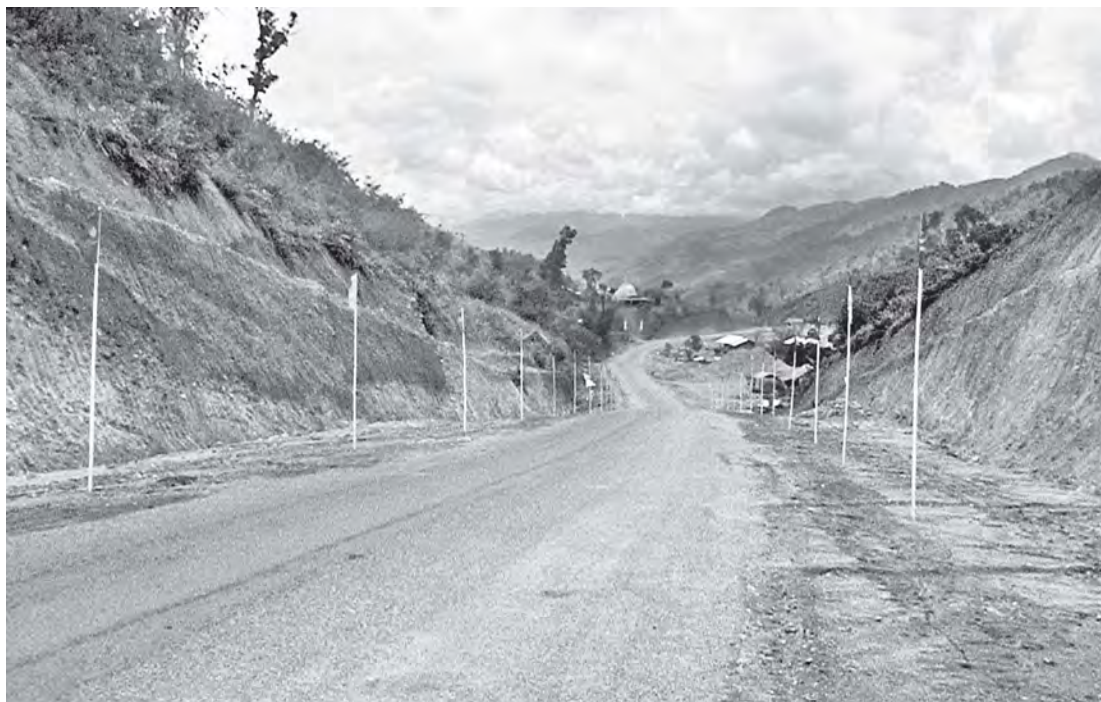
Photo shows a part of Nay Pyi Taw Pyinmana-Pinlaung (Kantha-Koegway) section asphalt road.
